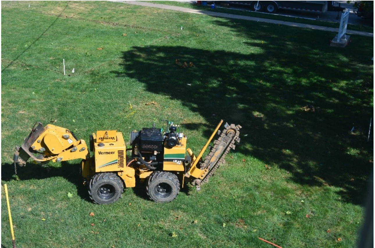
Irrigation system installation | Photo credit: Mary Osborne
